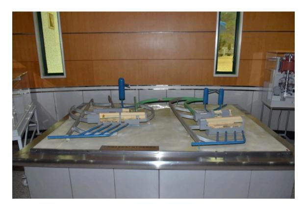
The turbines are reversible and can act as a power turbine when water is released from the upper dam and as a pump when under power to pump water from the lower to upper lakes.
